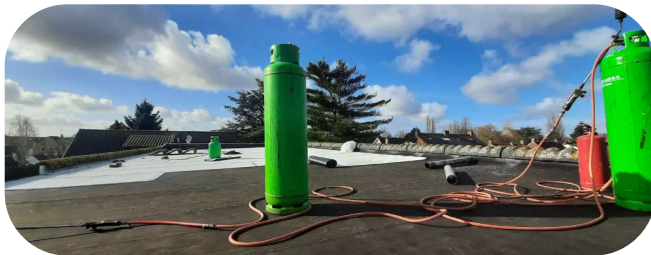
Flat roof resurfacing
